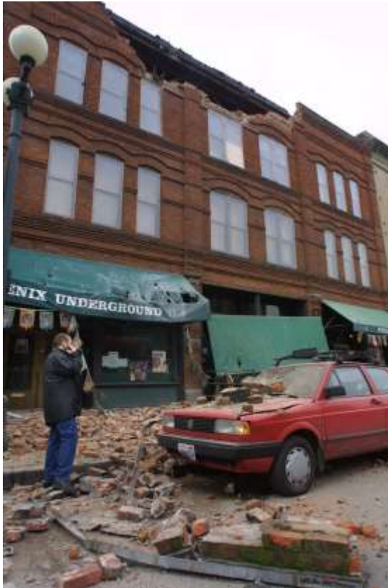
Nisqually Earthquake Seattle, 2001
