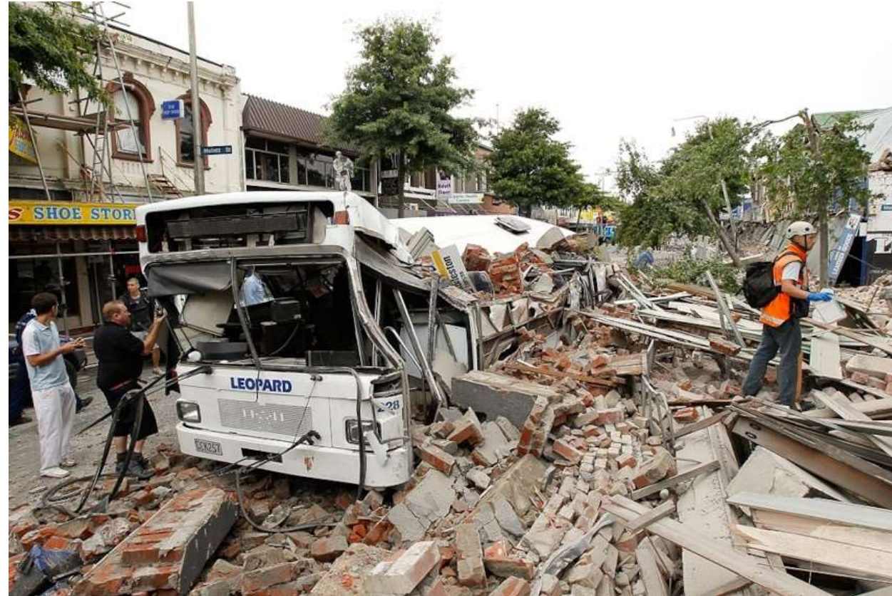
Canterbury Earthquake Christchurch, NZ 2011
